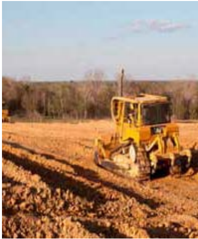
Site selection, pad site preparation
